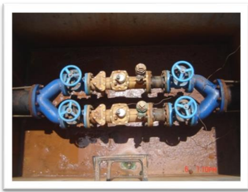
Meters at LaGrange Connection
