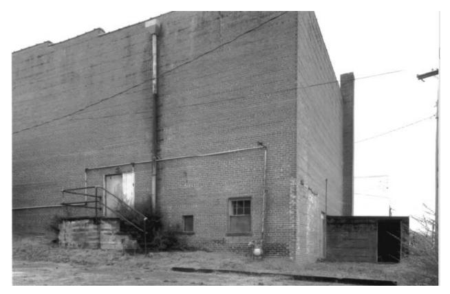
The photo of the rear of the building shows that the structure, which originally housed the cooling has been removed (far right), and that the low structure that remains housed the boilers. Other modifications include the removal of the exterior pair of doors at the top of the landing, which were replaced with a single door and infilled with wood.
