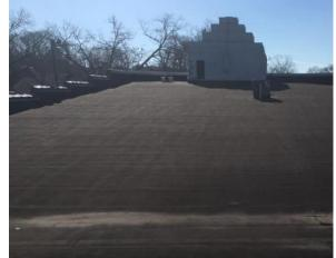
The photo at right identifies the first roofing problem: the drainage valley has very little slope (left to right) in order to direct water to the two scuppers.
