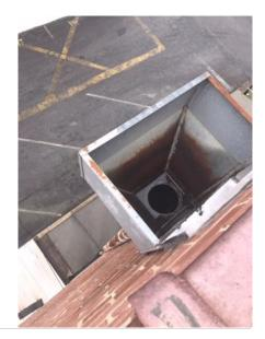
The existing roof leaks and likely areas of water infiltration include the original terra cotta parapet coping (left) and the through-wall penetration leading to the downspout collector box. However, based on the multiple areas of leaks and the age of the roll-roofing, it is suspected that the roofing joints or material itself has thematically failed.
