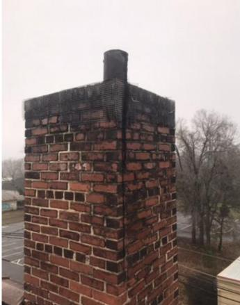
Boiler flue at left with wire to prevent rodents/birds from entering. Below is the collector box for one of the two roof gutters. The flue, which is no longer in use, enables water infiltration into the building. The collector boxes, which are not original, are inadequately sized and have rusted.
