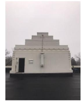
Exterior photos showing the restored masonry stucco which has held up well although there are some cracks that need addressing. Note the original tile wainscot is gone.
